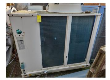
MODELLO .AQL 40.BFC.1P.PHC.3PH + N.FSC.C CE 1115 OdL 77926002 MATRICOLA SERIAL NUMBER 2771217918 ANNO DI COSTRUZ CARICA REFR. REFRIGERANT CHARGER ALTA PRESSIONE BASSA PRESSION 18.6 ALIM. POTENZA 3+N 50 CORRENTE DI SPUNTO 145 CORRENTE A PIENO CARICO 38.5 (max) A POTENZA ASSORBITA 20.1 PRESS. ESERC.ACQUA 3 MASSA (max) Kg 475 ITELCO INDUSTRY S.r.I Via XXV Aprile 29 200 MADE IN ITALY COD.0358
